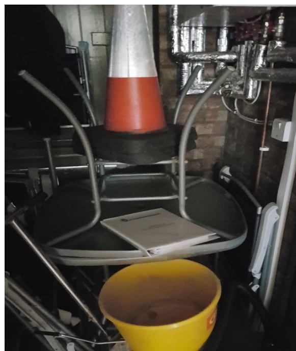
No.2 Relocate the combustible items to a more suitable location, away from direct contact with ignition sources.
