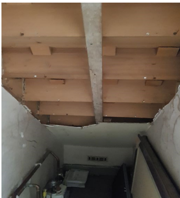
No.7 Underdraw with fire resistant plasterboard to a 30-minute fire resisting standard.
