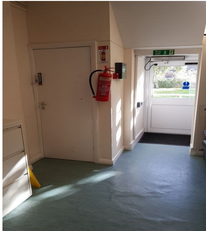
No.3 Display a fire action notice.
