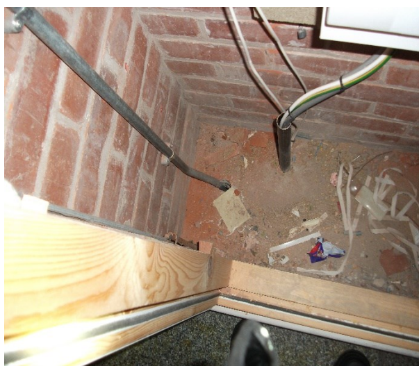
Cable penetrations in cupboard
