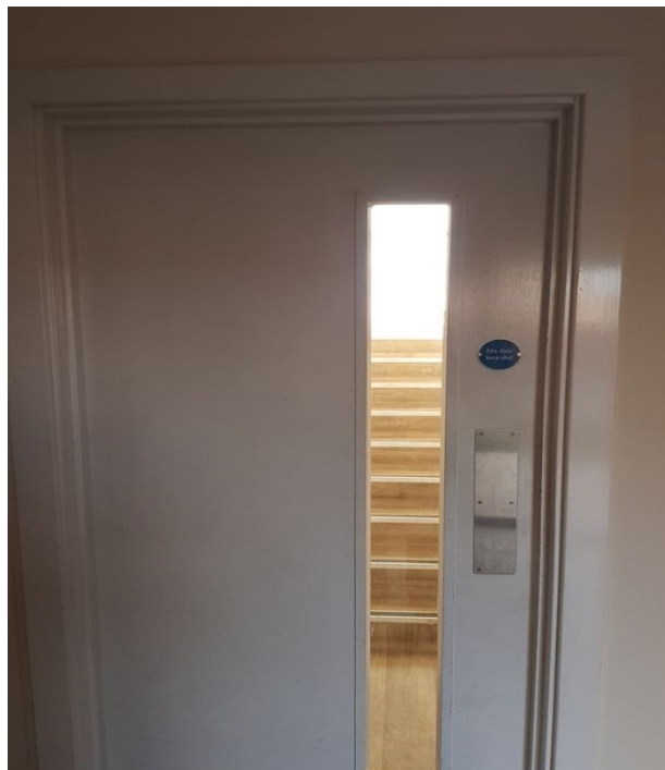
No.2 Replace the intumescent seals on all floor levels with intumescent smoke seals (stairways).
