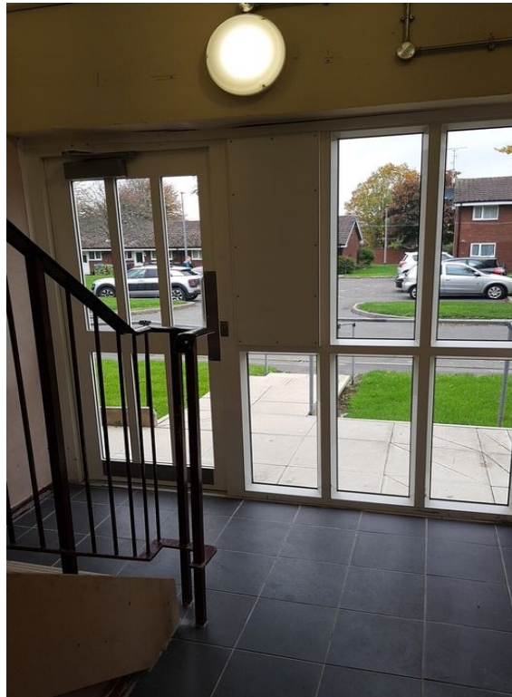
No.3 Display a Halton House specific fire action notice.
