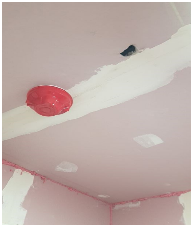
No.4 Remove the dust cap from the smoke detector.
