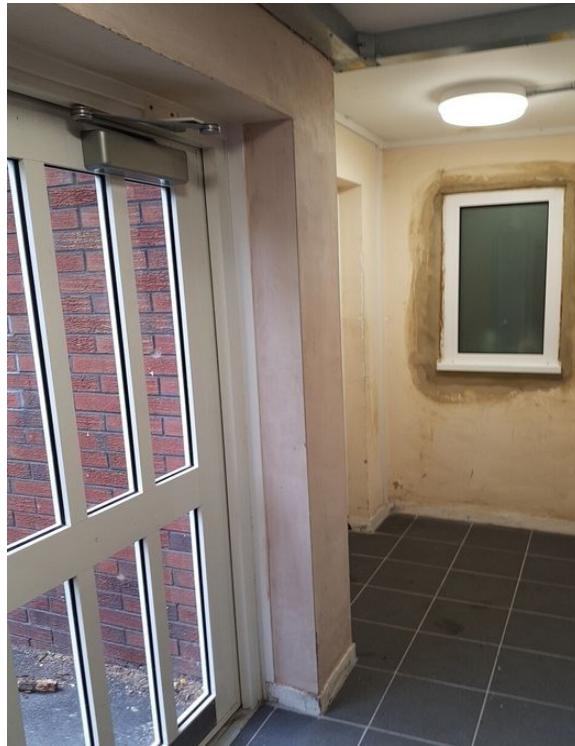
No.3 Display a Halton House specific fire action notice.
