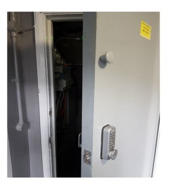
No.1 Intumescent smoke seals should be incorporated in to the electric meter cupboard door or frame
