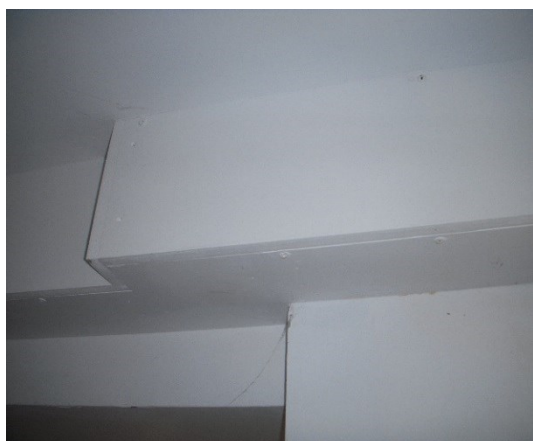
Timber boxing over electrics in common areas.
