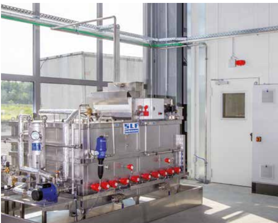
Process water treatment system for a cleaning booth
