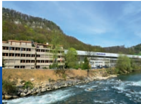
HAEUSLER headquarters in Duggingen, Switzerland
