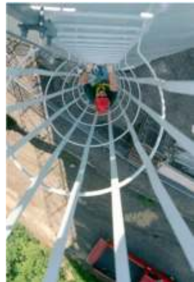
A worker using a vertical lifeline and ladder system to provide maintenance on a water tower.
