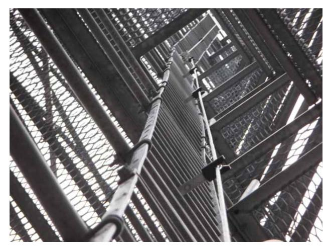
Vertical Lifeline Systems allows movement up and down the entire height of the line, eliminating the need to disconnect and find new tie-off points while ascending or descending from applications like a tower or ladder. By connecting to the vertical lifeline using a deceleration device, users may move as long as tension is slack on the lifeline.
