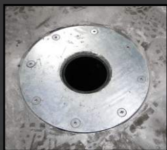
Installed Flush Floor Mount Sleeve Pt# 50042
