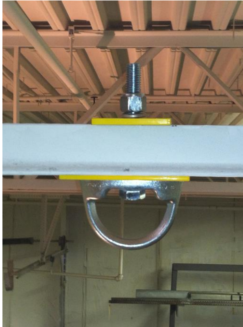
Figure 10 - Proper Assembly of FTA
