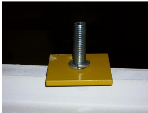
Figure 8 - Split Washer on Assembly
