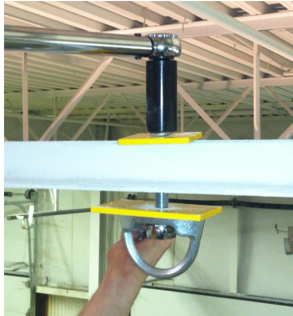
Figure 18 - Torque Lock Nut to 75 ft-lb
