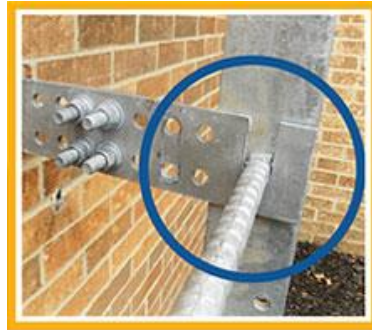
2 Place rung in bracket
