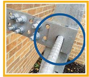
3 Secure with bolt-on capture plate
