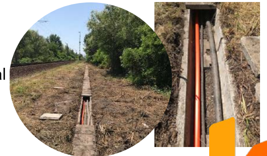
Microduct - Direct Buried, Direct Installed Duct Example ) 14/10mm 7way + Micro cable 144 Core * 7 tubes (1,008 Core) 16/12mm 7way X Micro cable 432 core * 7 tubes ( 3,024 core)
