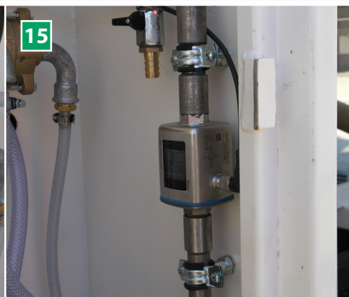
15 Flow measurement chemistry (optional) Electromagnetic flow measurement, 1/2" in stainless steel, max. 16 bar, temperature -10 to +70 °C, minimum conductivity 20 µS / cm. The flow measurement guarantees a dosing accuracy to +/- 2 % (repeatedly +/- 0.2 %), according to EN 206-1.
