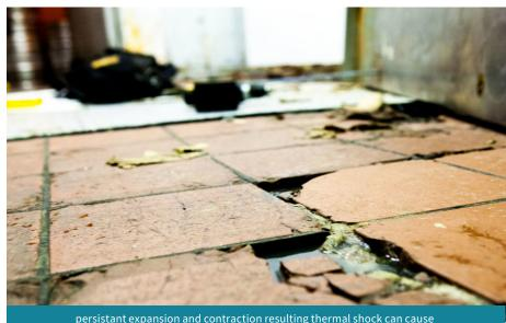
persistant expansion and contraction resulting thermal shock can cause tile grouts to fail and seperate
