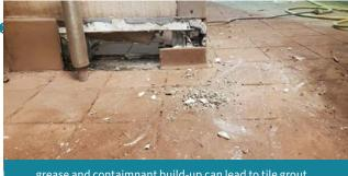
grease and contaimnant build-up can lead to tile grout failures and eventual delamination
