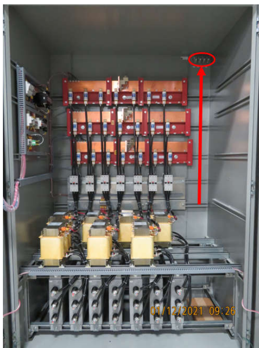
Figure 6.3 Safety Ground Connection. See table 6.2 for torque specification
