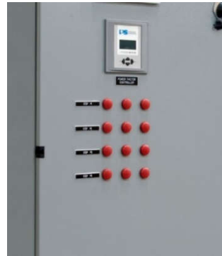
Figure 7.4 BFI will illuminate when fuse is blown (open)
