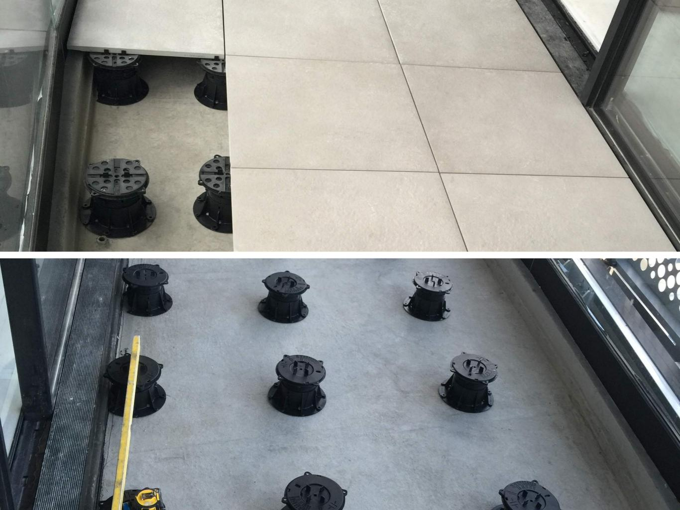
The Buzon DPH pedestal system solved this, not only accommodating the variable heights and slopes, but also the odd shaped pavers and curves. Within the radial area of the project, BC pedestals were installed under pavers utilising the circular tabs to achieve the curve, creating a stunning feature in the atrium.
