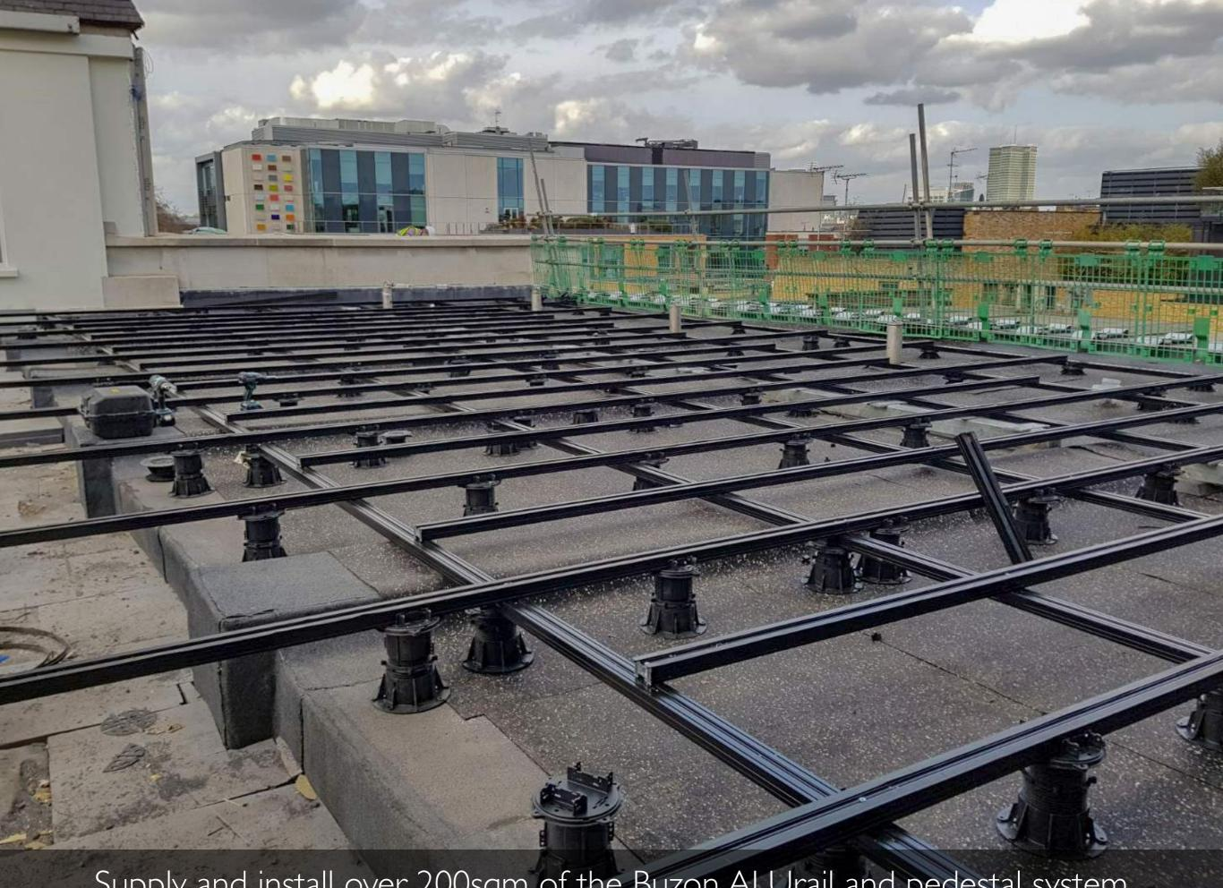
Supply and install over 200sqm of the Buzon ALUrail and pedestal system
