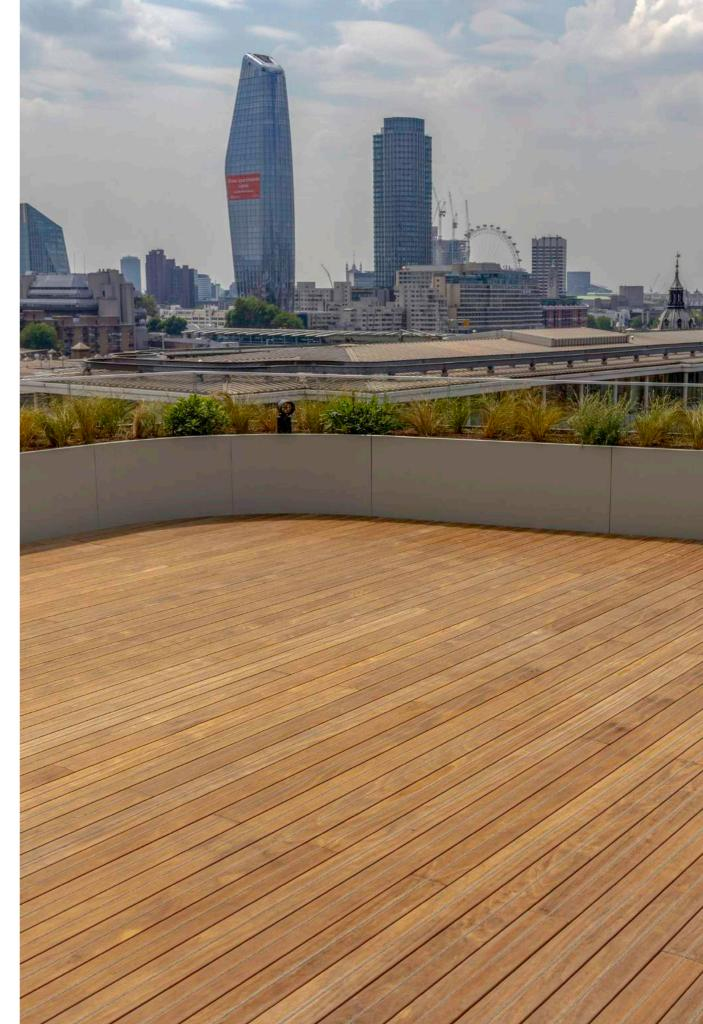
Buzon UK were commissioned by Frost Landscape Construction to supply and install the DPH pedestal system to support GRAD decking and rail systems supplied by the Outdoor Deck Company.
