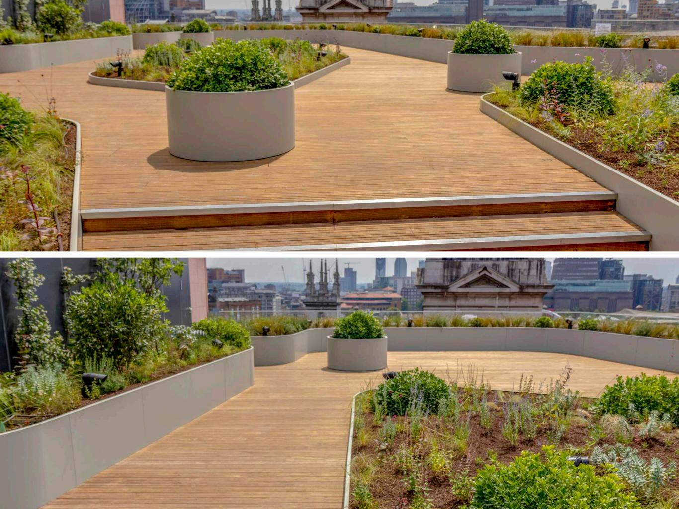
This was a particularly challenging project as powder coated steel planters were strategically located in the middle of the roof terrace so the installation of the adjustable support pedestals had to be carried out around the numerous planters
