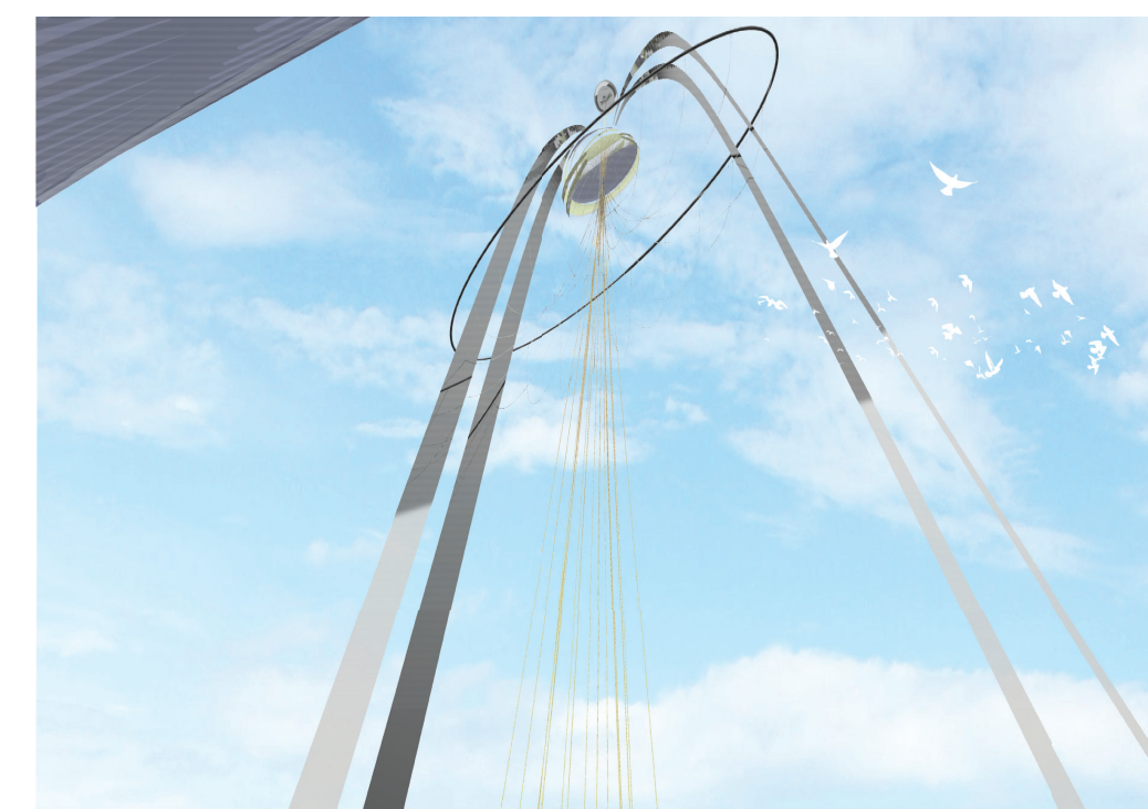
The light tower is a carbon-steel structure stands 170 ft tall that can be seen within 8 miles radius.
