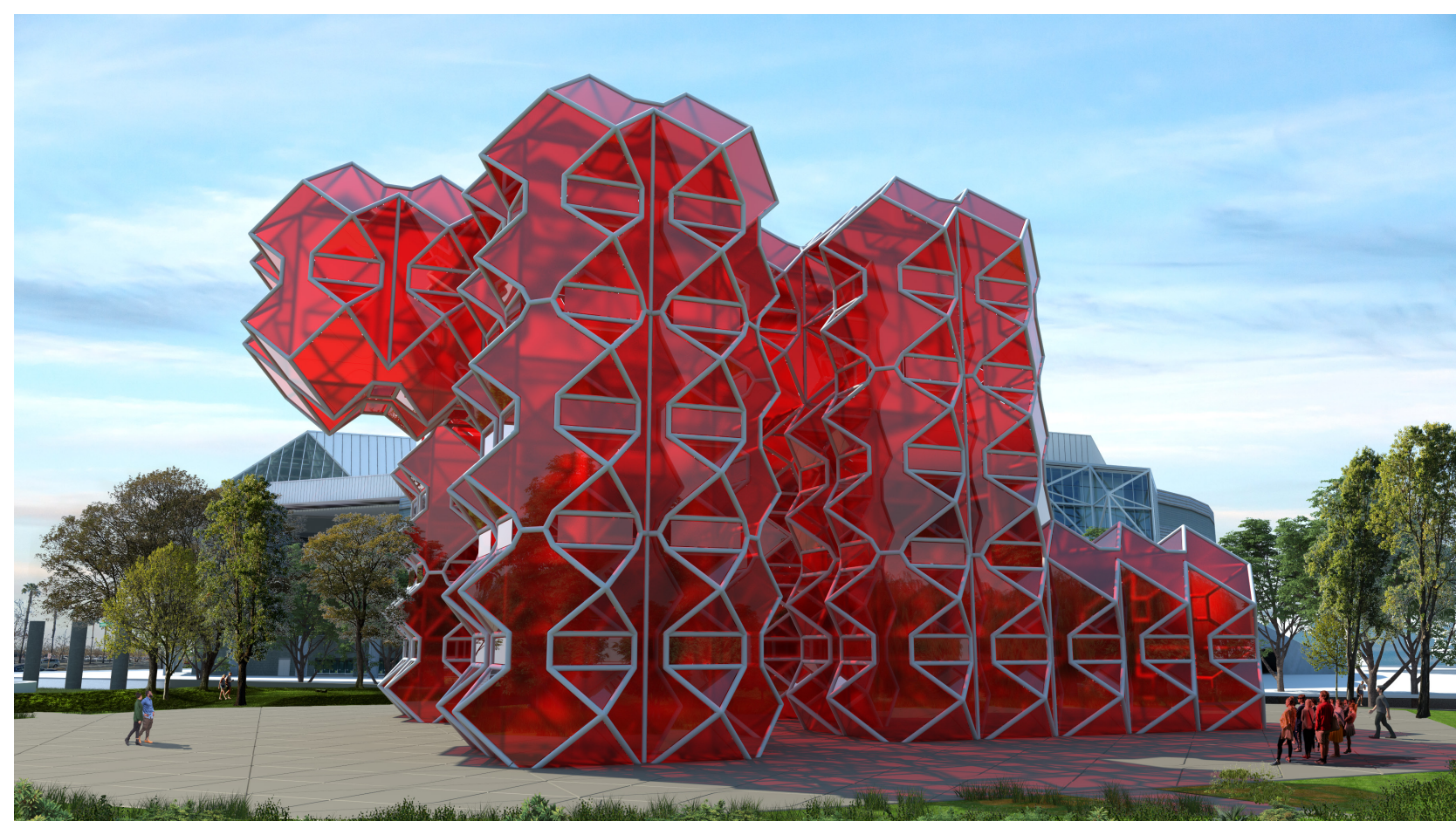
The Red Giant is a sort of huge iconic semitransparent portal that the public can cross. The light that passes through the structure paints the area and passers-by who walk near the sculpture.
