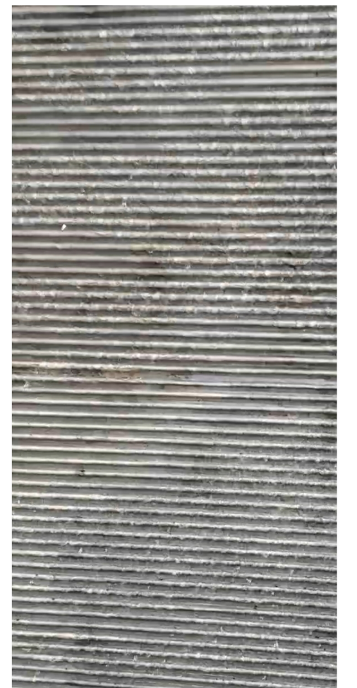
Exterior walls are ridged to keep water flow uniform
