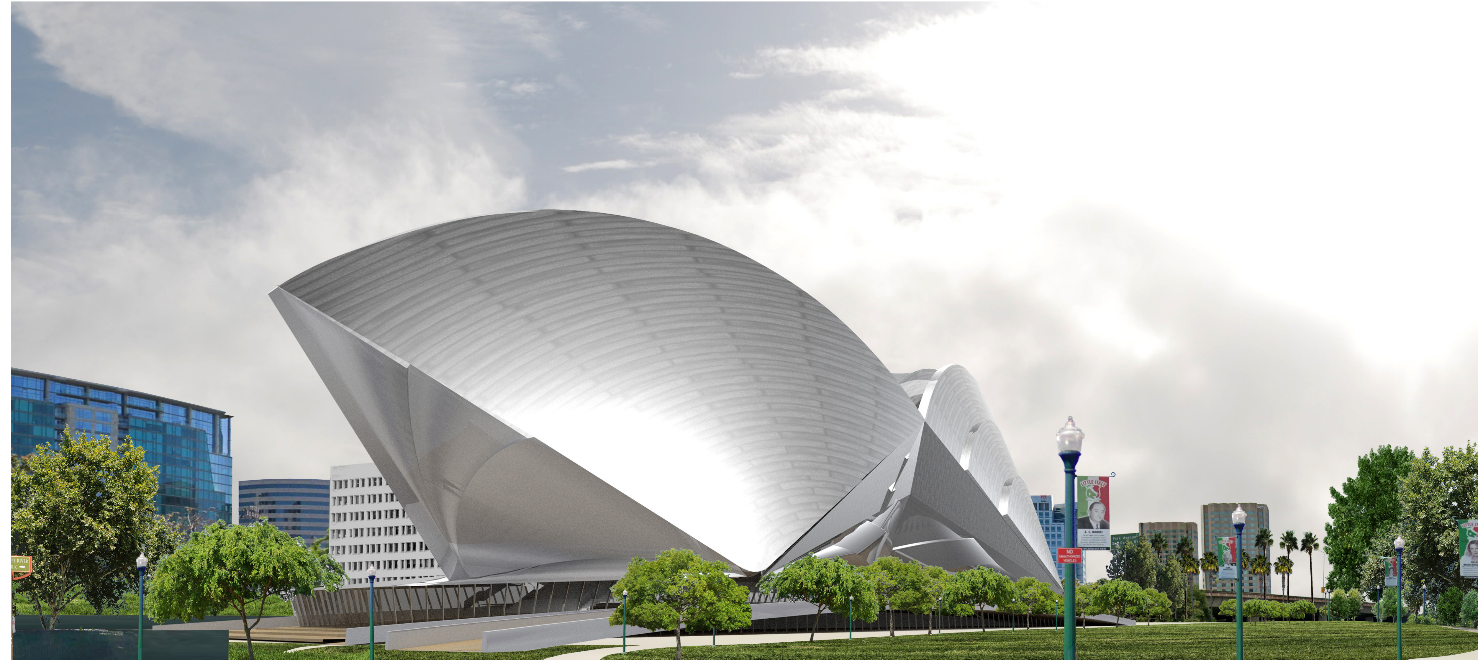
View from North at St John Street
