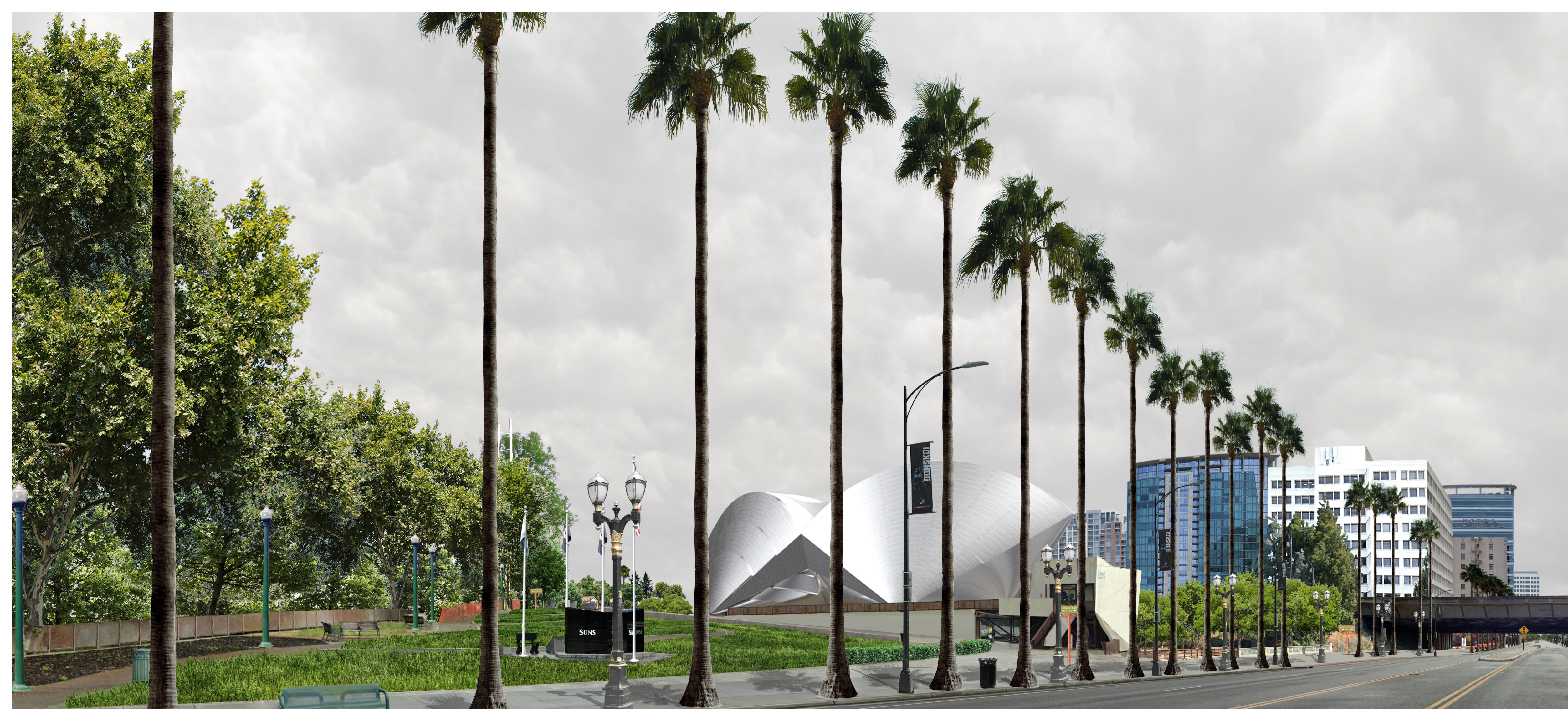
View from West at the Santa Clara Street
