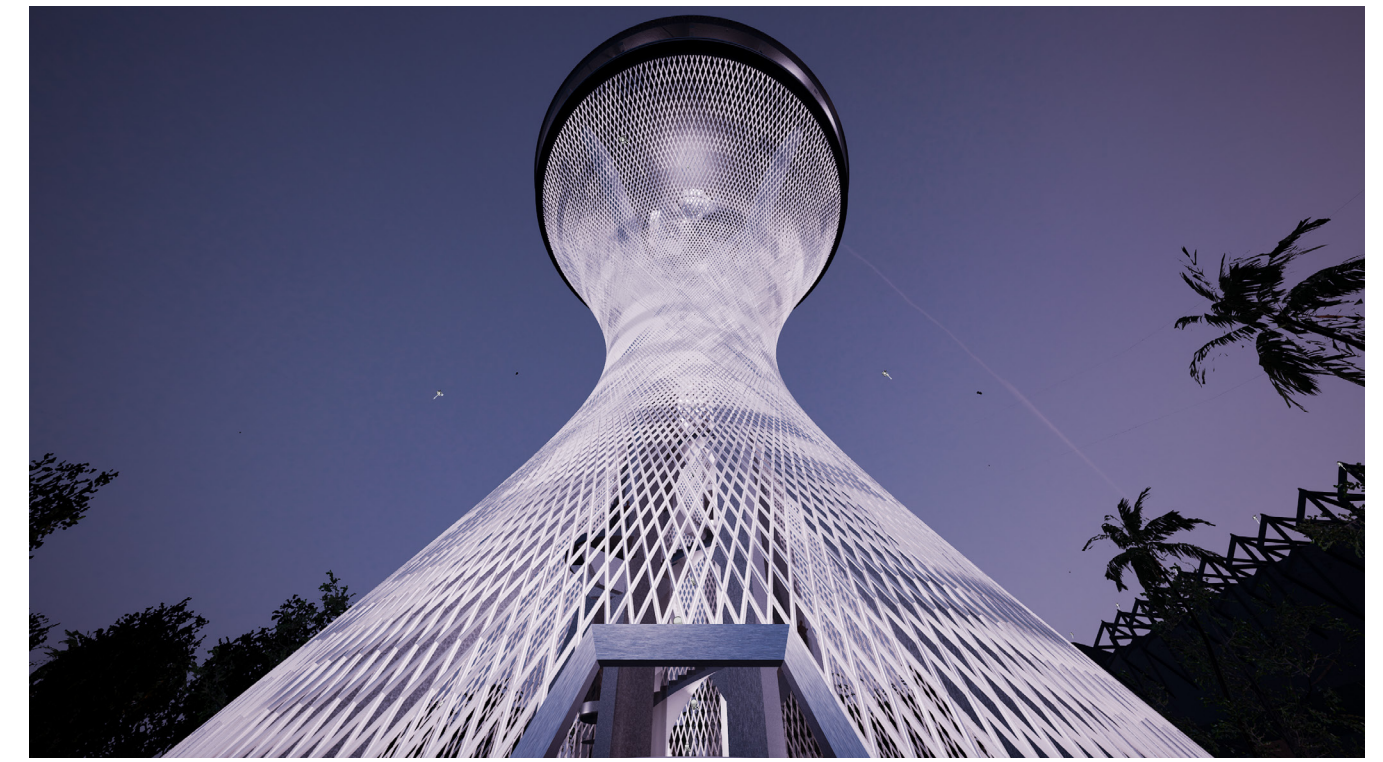
The mesh is a hyperboloid display with 4 million light pixels
