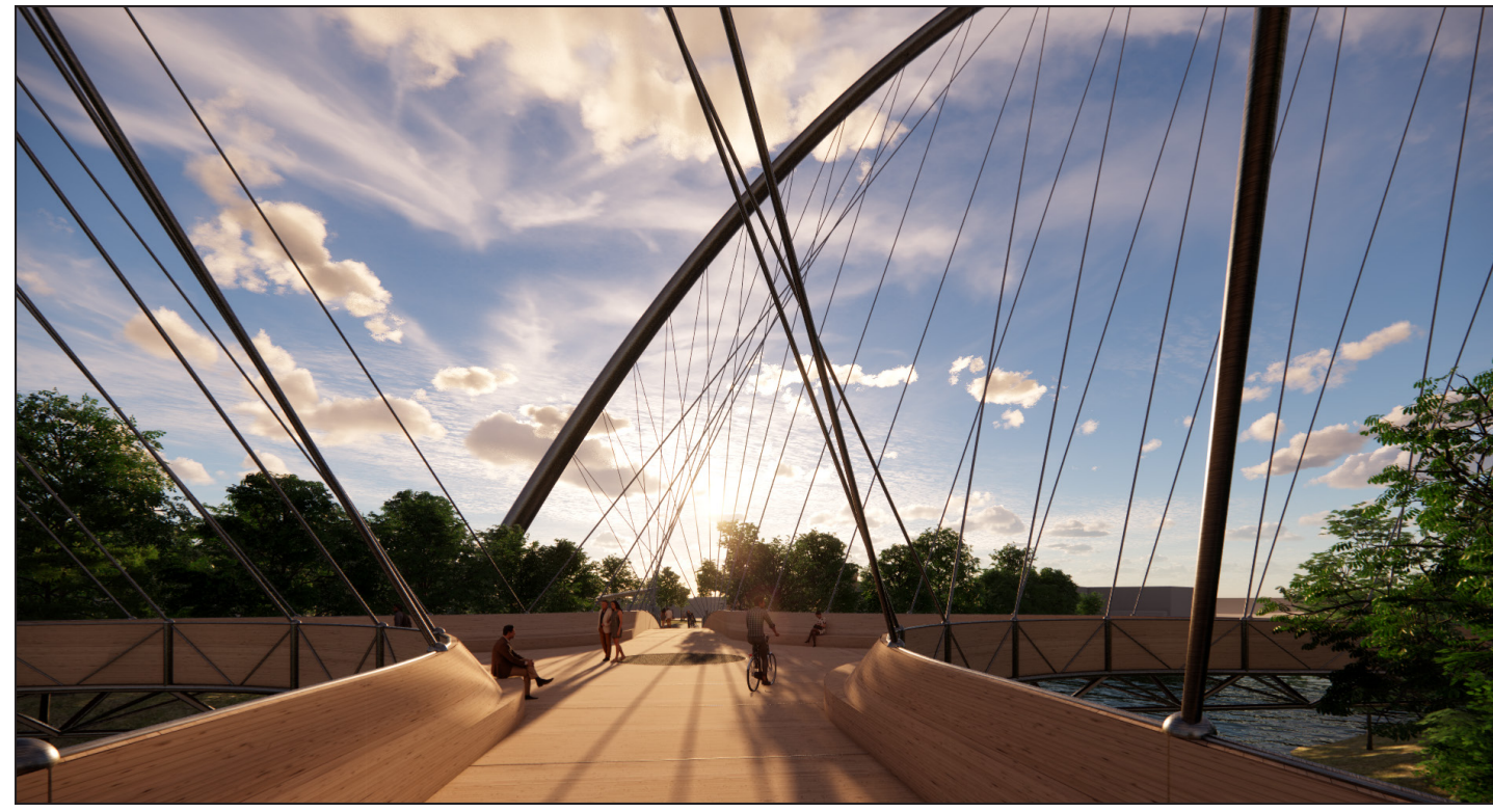
The Intersection. The center of the bridge is an exciting place, converging above the river (which is itself converging). It manages bike and pedestrian traffic around the center, which is a grated port to the river below. Built-in benches encourage reflection and recline to look up at the harps above.
