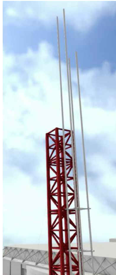
Figure 12-7: Each sub-assembly is then rotated into the vertical position by a series of cables rigged from a hoisting tower.
