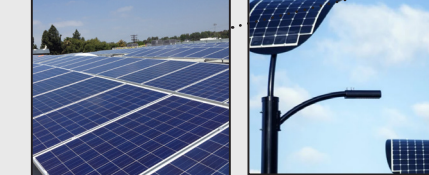
Solar array solar powered, tectonic lighting activated by motion sensors to protect aviation and fauna from disturbance.
