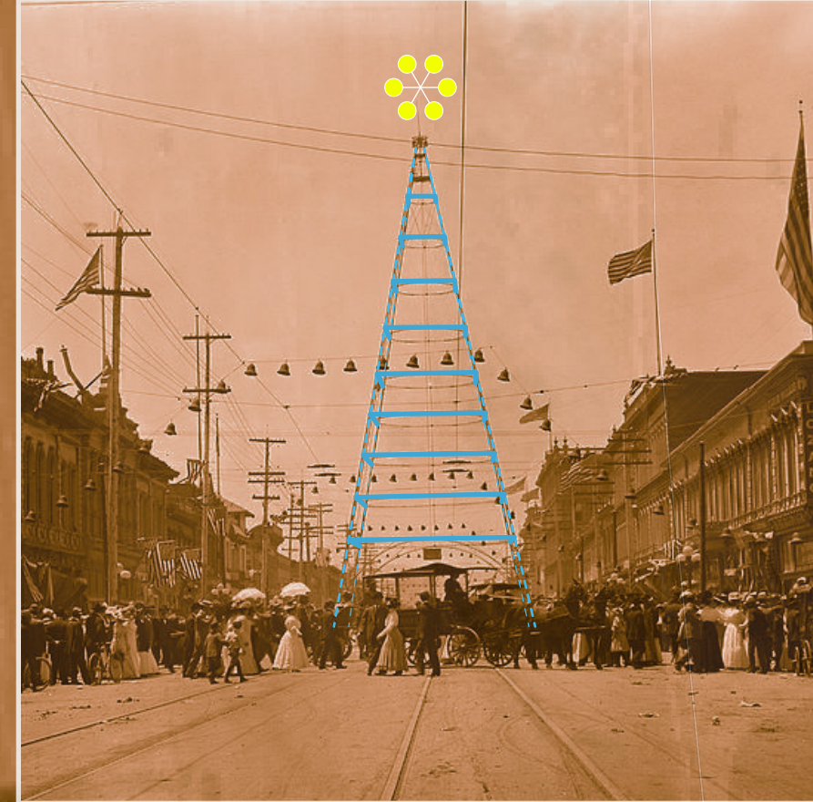
Original San Jose Light Tower
