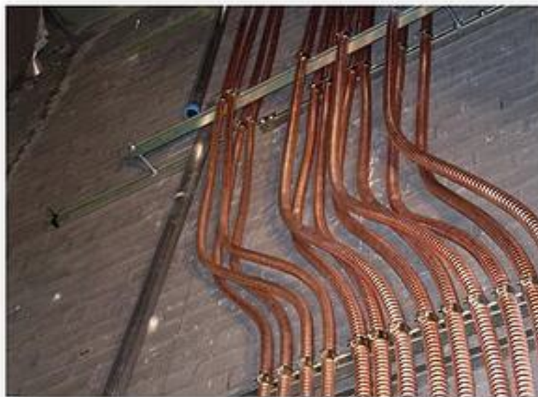
Fig. 7) VITALink® MC Tested and approved to run vertically
