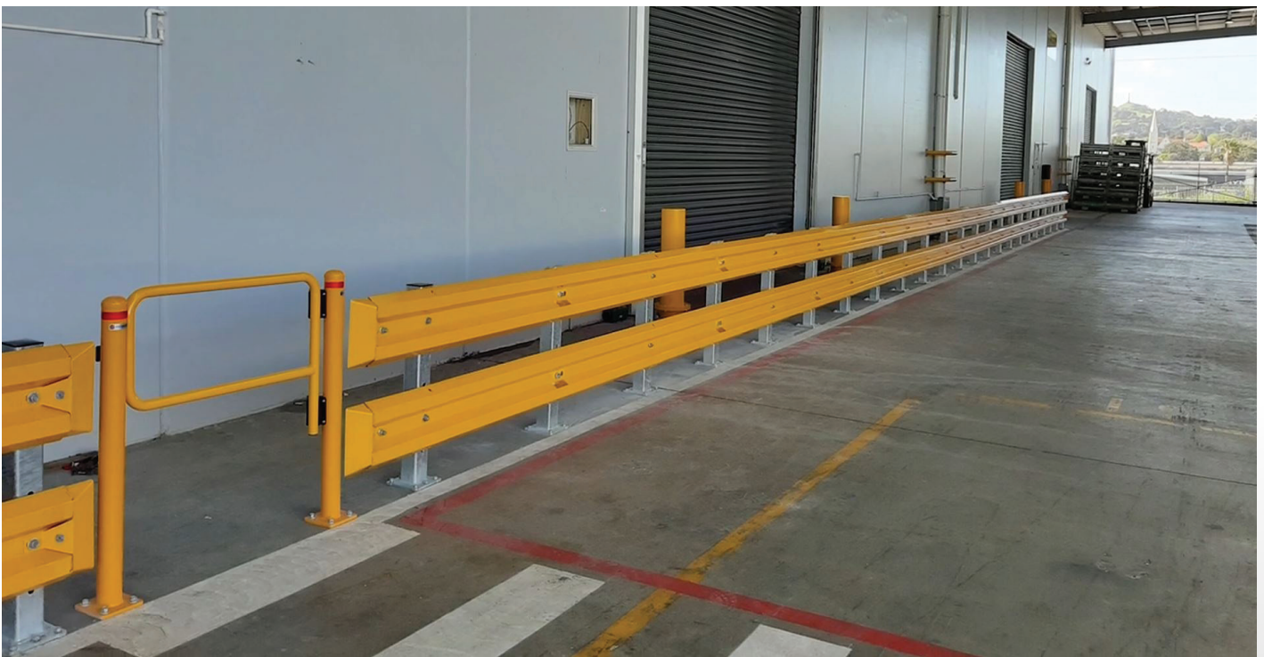
Pedestrian and vehicle management system next to loading zone.
