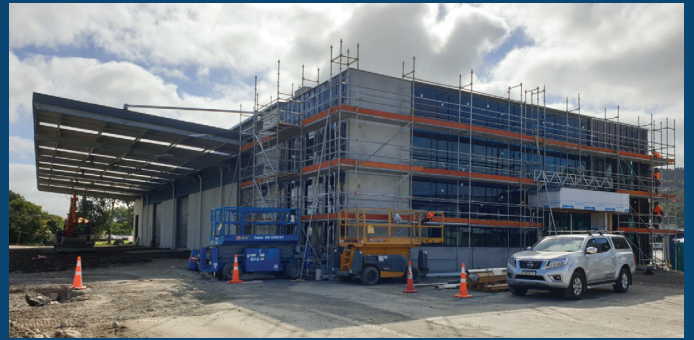
New Vanguard warehouse in construction.
