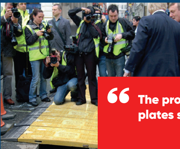
Road Plates being used to cover trench
