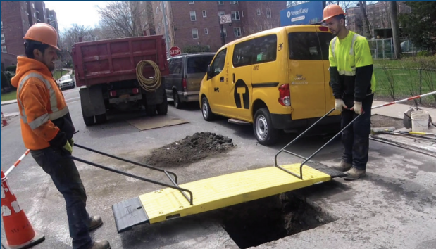
Road Plates being installed with assistance device
