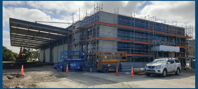
New Vanguard warehouse in construction.
