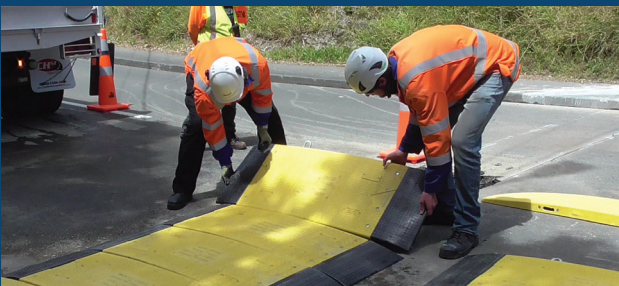
Road Plates being used to cover trench
