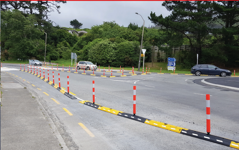
New traffic management system, temporarily directing vehicles
