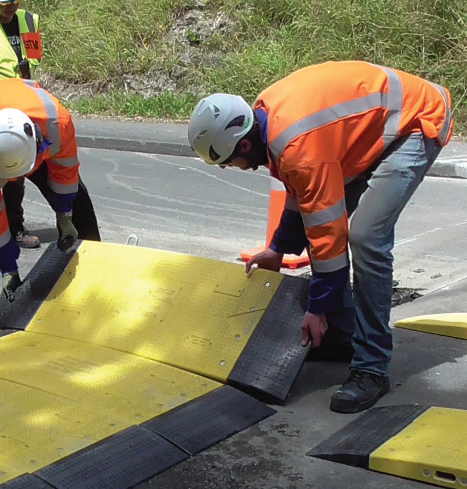
Roadworkers laying new fibreglass Road Plate
