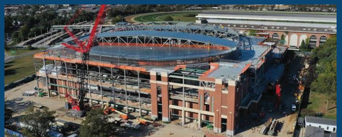
UBS Arena under construction in New York
