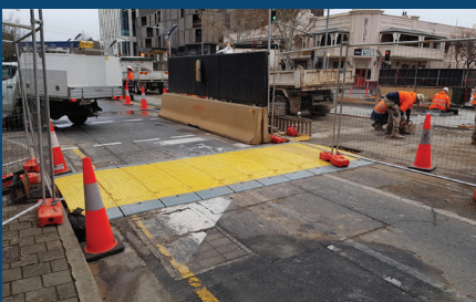
Anti-slip and hi vis surface
