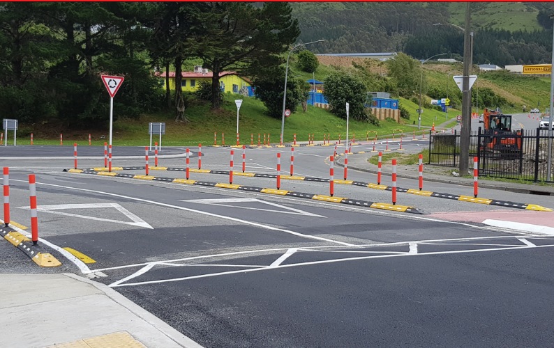
Traffic Separator system at Porirua intersection
