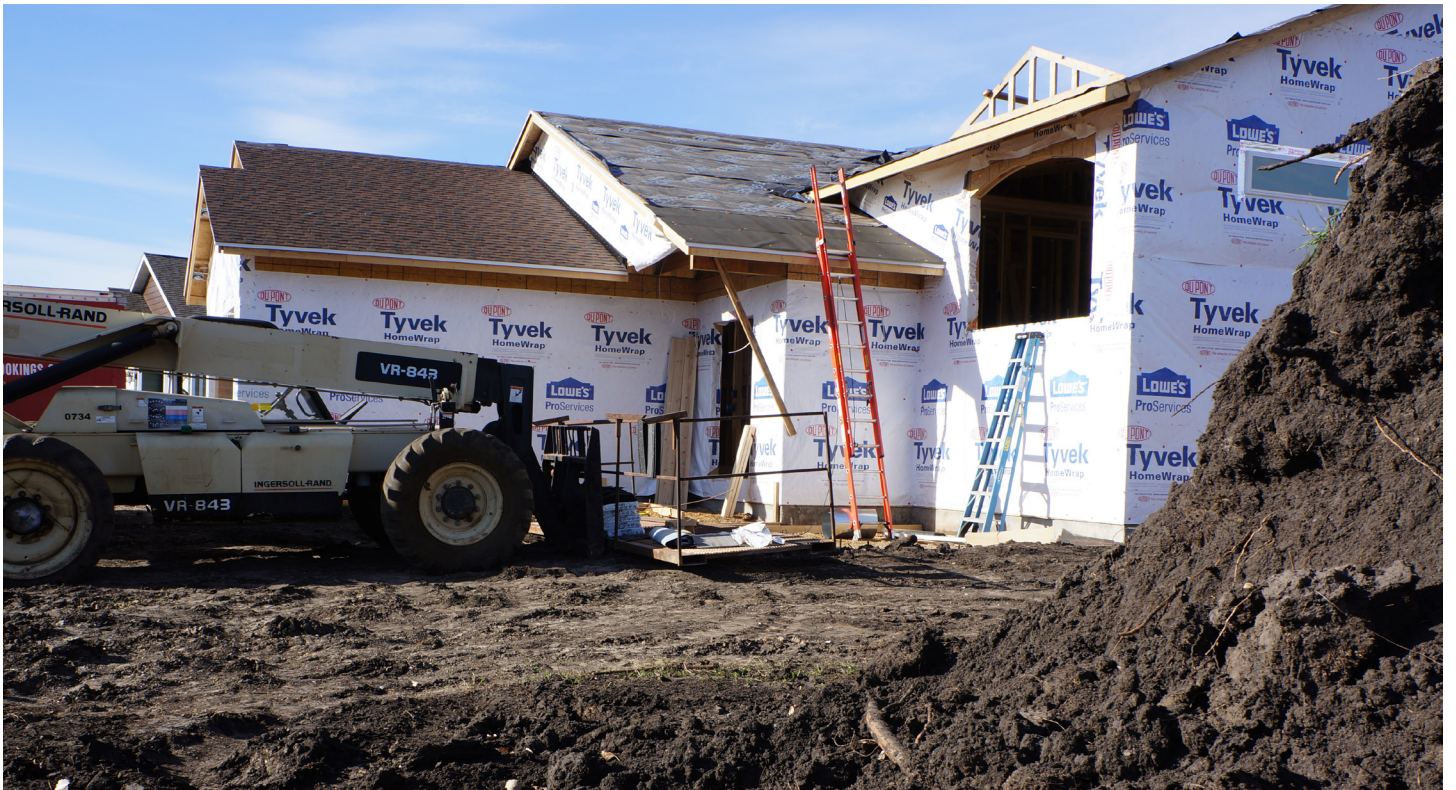
CJ & Jill Knutson's New Construction Project in Process
