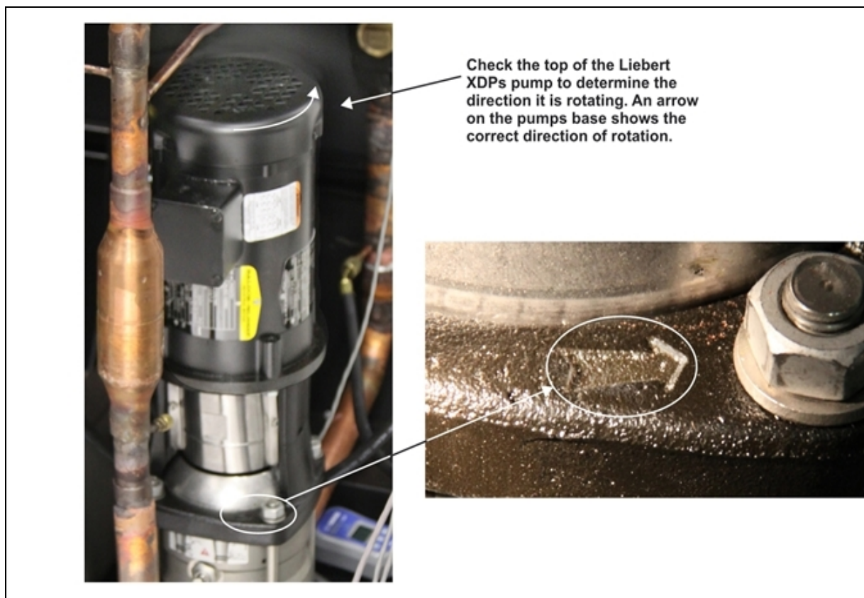
Figure 5.1 Liebert XDP pump rotation determination
