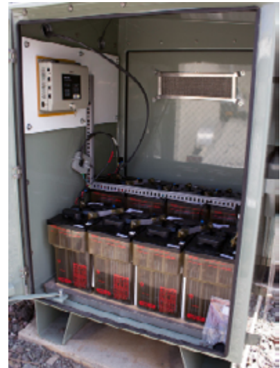
Installation to 48V Switchyard Battery
