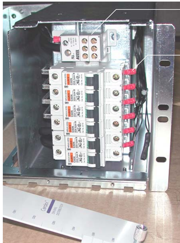
Figure 5—DIN-type circuit breaker distribution module with cover removed
