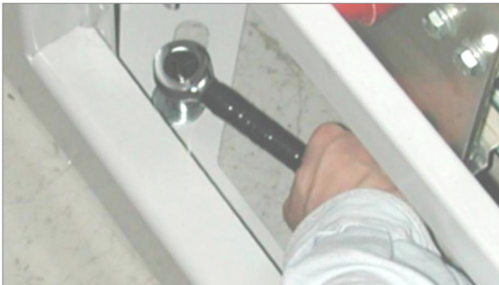
Figure 29 — Securing Power System to Concrete Floor
