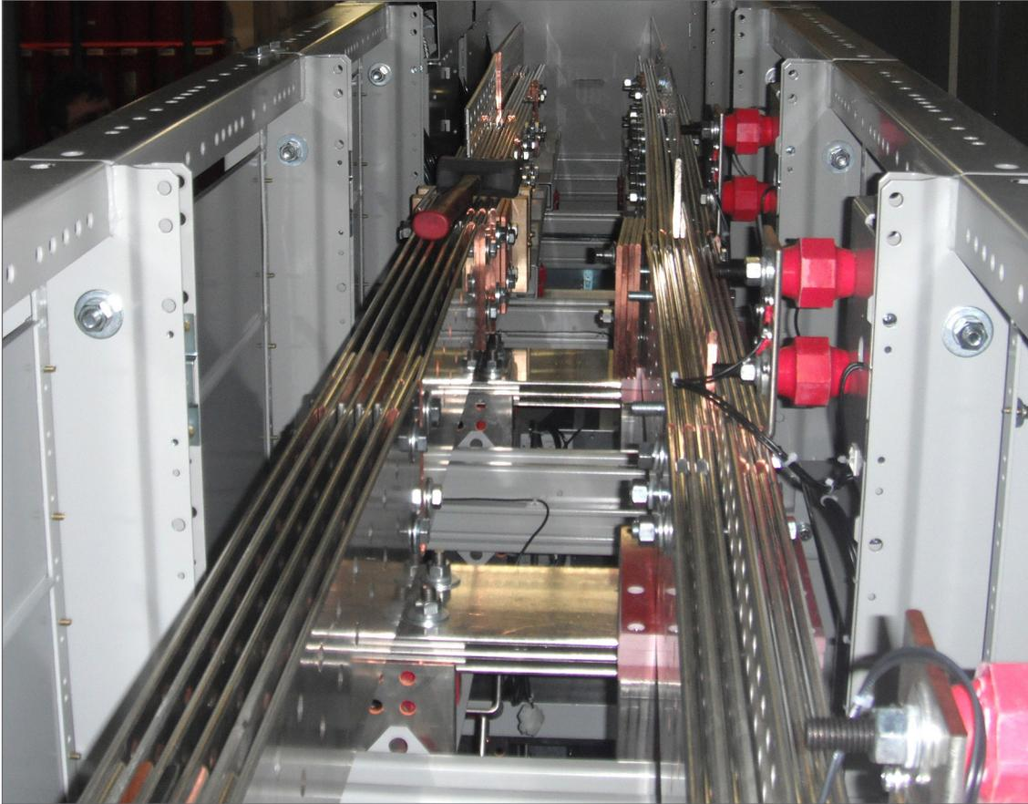
Figure 31 — Example of Installed Inter-bay Buswork
