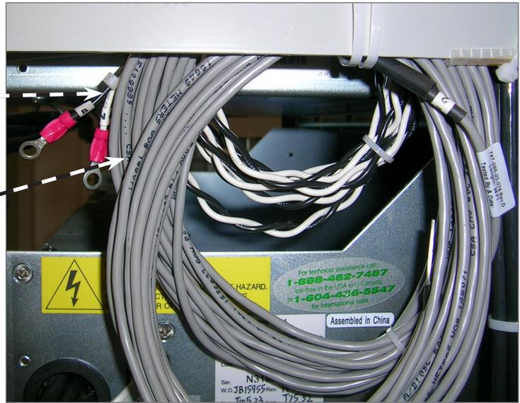
2. Connect current shunt leads. Refer to Figure 20 for the location of the shunt in the distribution bay.
