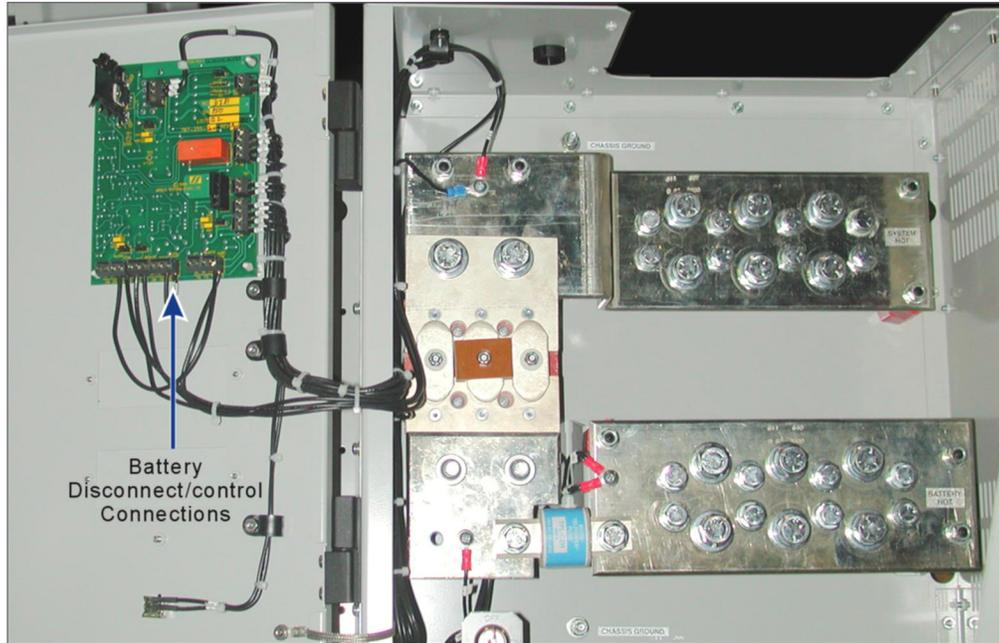
Figure 39 — Battery Disconnect Connections
