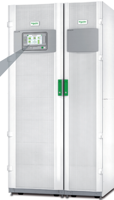
UPS with input/output cabinet
