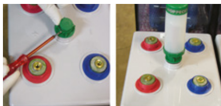
Fig. 5-14: Labyrinth plugs (left) and grid | aquagen recombination system (right)
