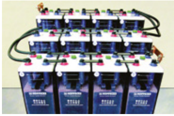
Fig. 5-16: Using row connectors and step connectors
