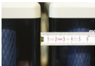
Fig. 5-13: 10 mm clearance between the batteries
