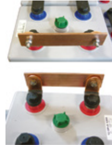
Fig. 5-18: Installing the end terminals (connection plates)
