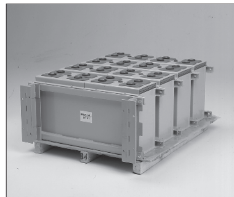
I-BEAM SUPPORT INSTALLED Figure 8
