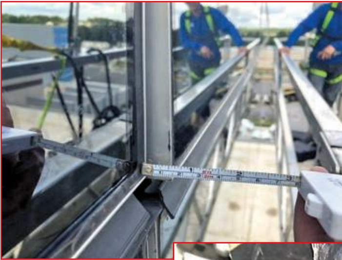
Figure 6 – Partially unengaged glass slab edge cover.
