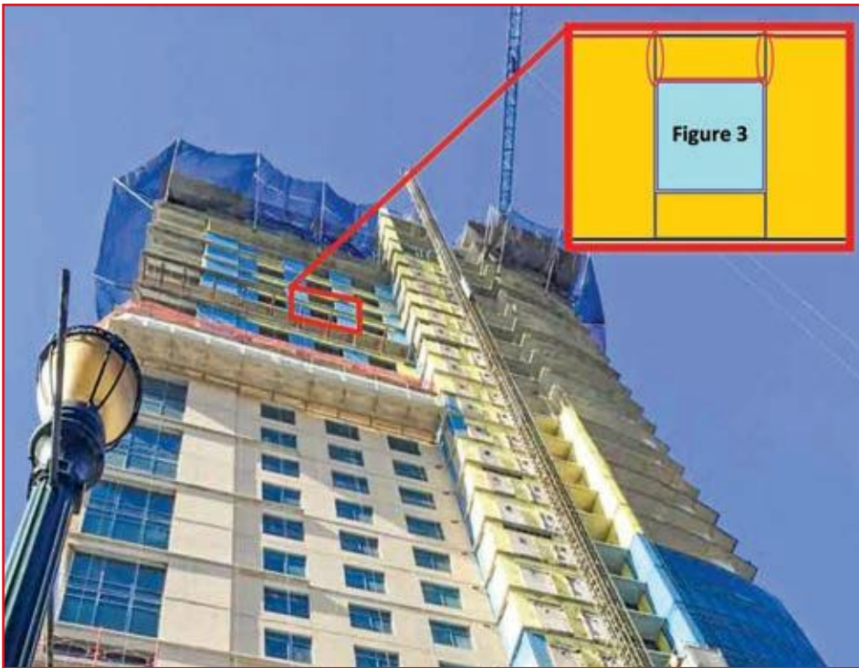
Figure 2 – Prefabricated panelization of exterior wall system.
