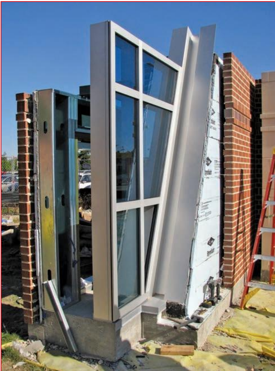
Figure 14 – Independent phased field mock-up of exterior wall and fenestration transitions.
