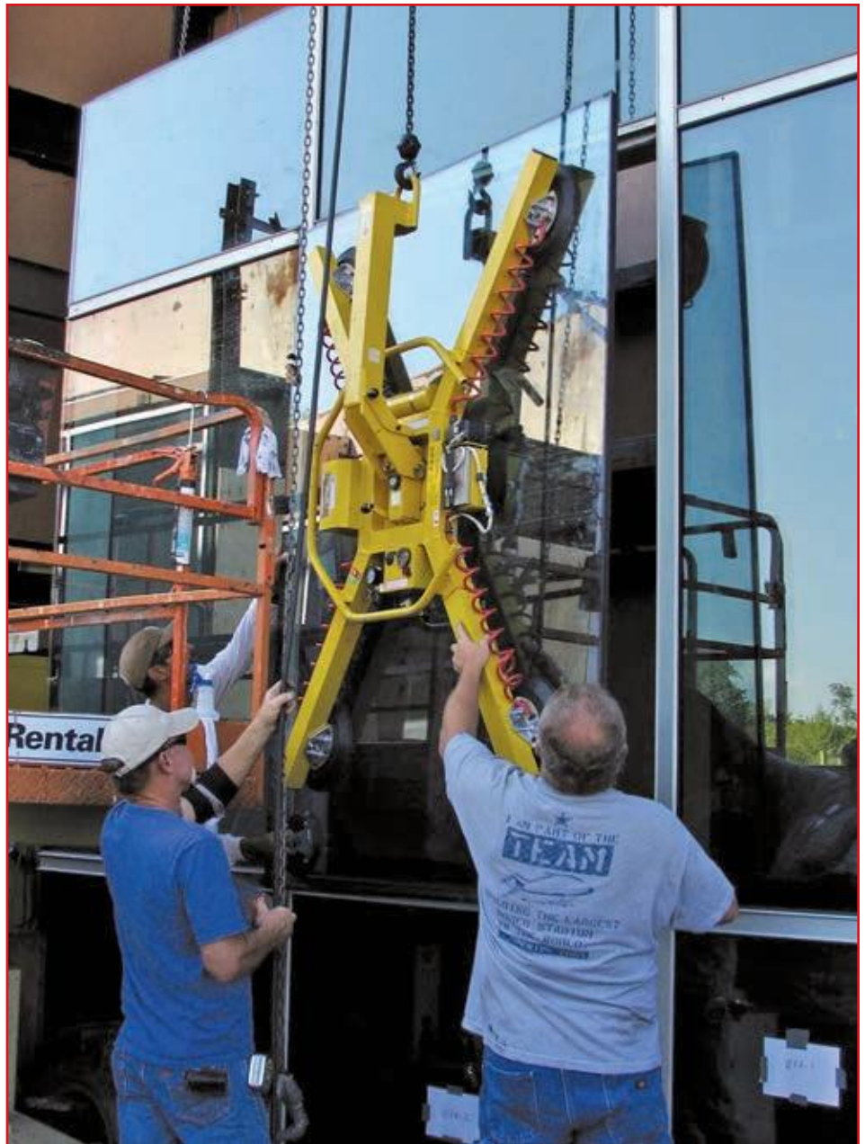
Figure 13 – Re-glazing at preconstruction mockup test specimen.
