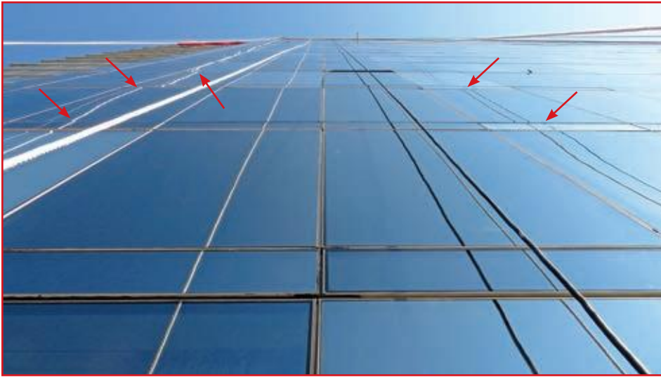
Figure 9 – View looking upward along elevation. Note non-uniformity in reflection of lifelines and power cord from floor to floor.
