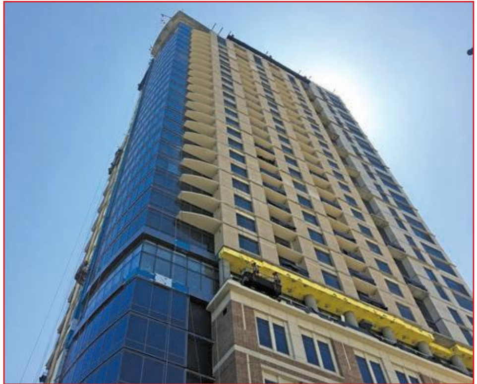
Figure 1 – Luxury residential high-rise, view of northwest corner during construction.
