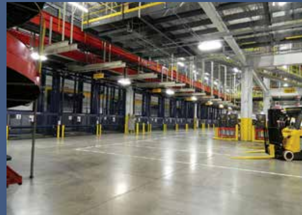
Distribution Center Material Lifts – F Series Mechanical VRC Global logistics distribution center relies heavily on 20 high-capacity VRCs with state-of-the-art sorting capabilities. 15,000 lbs. lifting capacity per lift.
