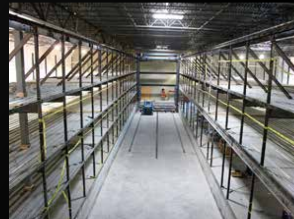
Robotic Parking System – High-Speed Vertical Lifts 7-level, high-speed vertical parking garage stores 325 cars. Programmable controls ensure uninterrupted operation. Lifts send and retrieve automobiles at a rate of 400 FPM.
