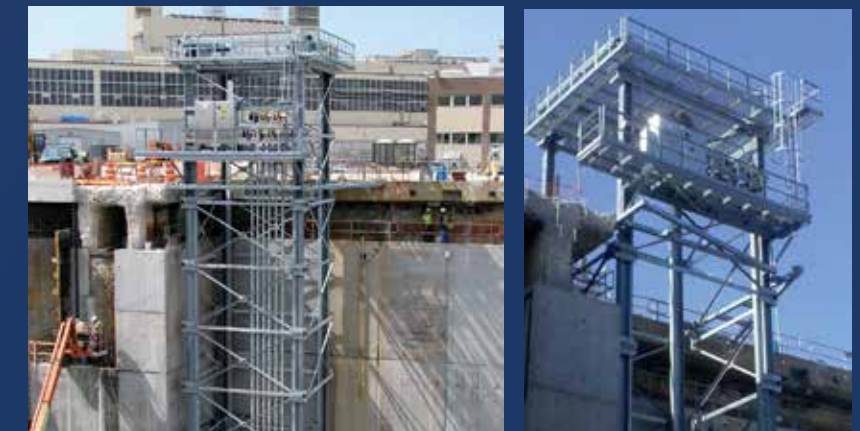
Naval Shipyard Drydock – F Series Mechanical VRC High-capacity lift moves materials and equipment used to build, repair and modernize the Navy's largest ships. 30,000 lbs. lifting capacity; 50' lift travel; 30' per minute travel speed.
