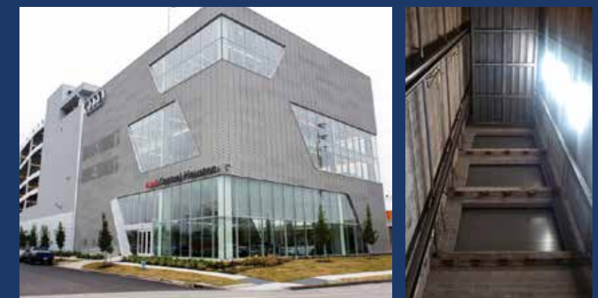
Auto Dealership High Rise Lift – F Series Mechanical VRC High-capacity lift moves luxury automobiles to storage and service levels. 8,000 lbs. lifting capacity; 73' lift travel; 6 levels of service.
