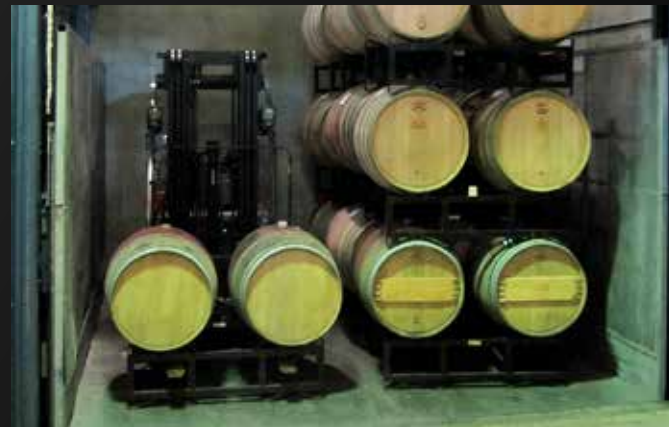
Winery Lift – F Series Mechanical VRC This through-floor application is in service year-round, and in constant use 12-14 hours each day. 20,000 lbs. lifting capacity; 26' lift travel; 3 levels of service.
