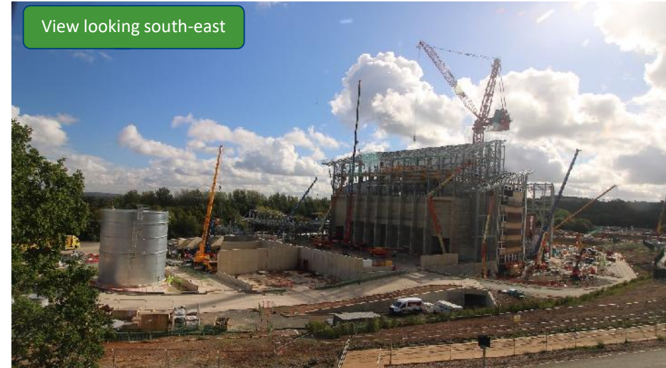
Boiler Panel installation
