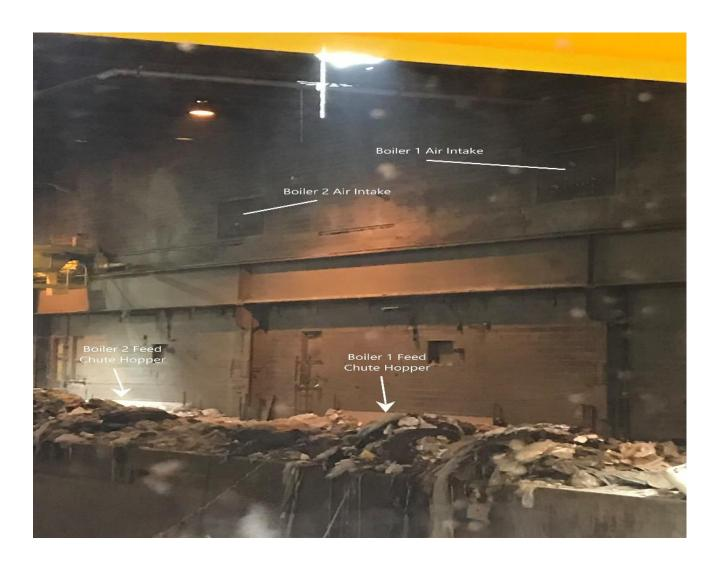
**Photo # 3.** View from tipping floor illustrates vertical nature of vent relative to tipping floor, pit and charging hopper. Any gas from those areas is drawn to the vent. Monitor located below the vent would have potential to be exposed to all gases including iodine gas.
