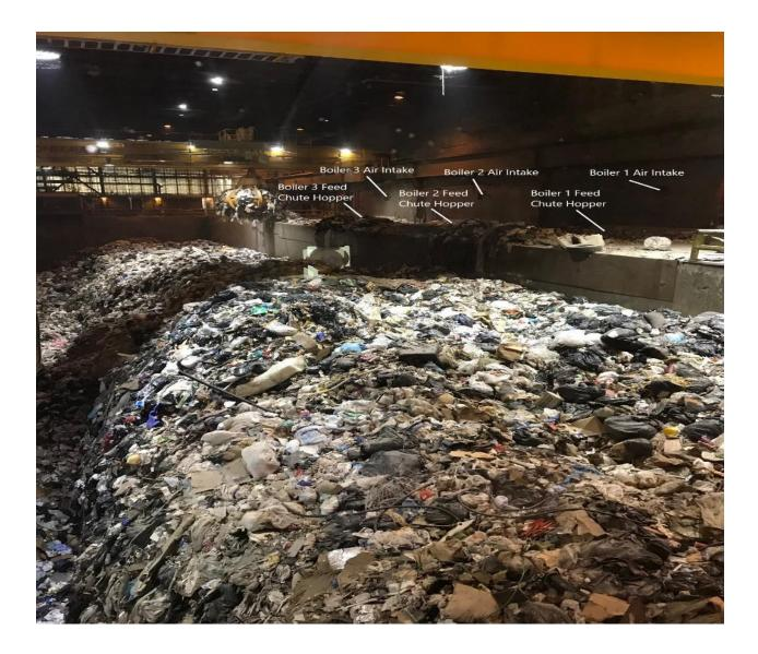
**Photo # 2.** Close up view of the furnace charging hoppers in relation to the air intake vents.
