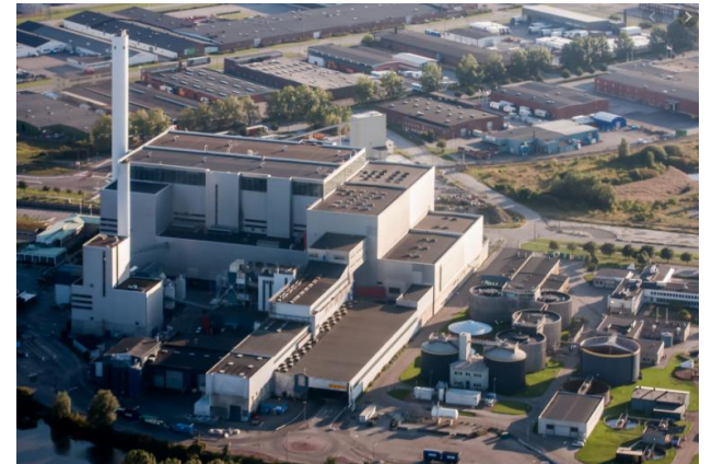
SYSAV WTE Facility in Malmö, Sweden
