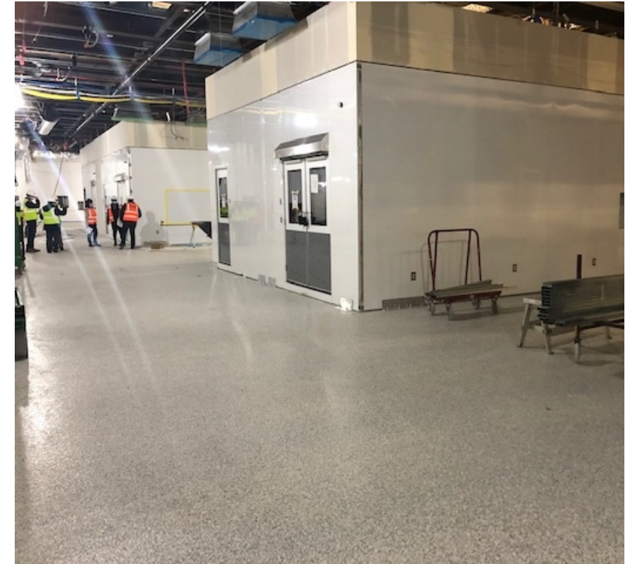
PODs moved into place
