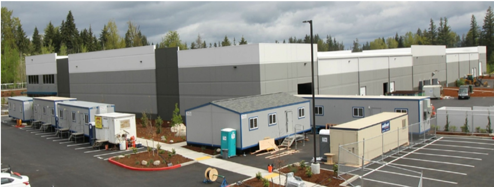
View of Building Shell Exterior
