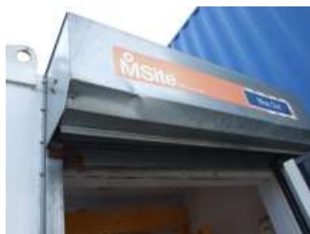
Dent to Roller Shutter
