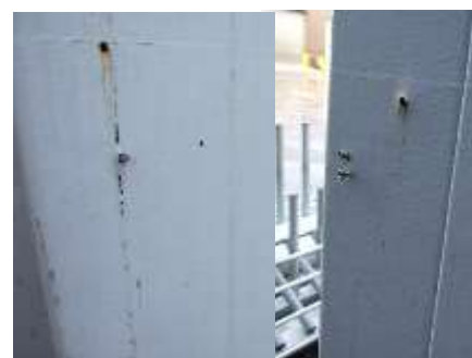
Bolt holes inc screws and bolts attached
